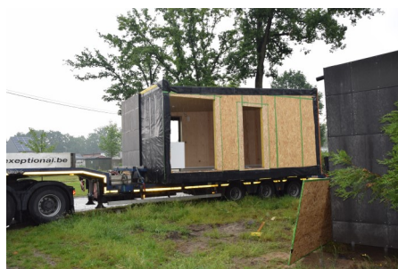
Modular homes at the Rustenberg pilot
